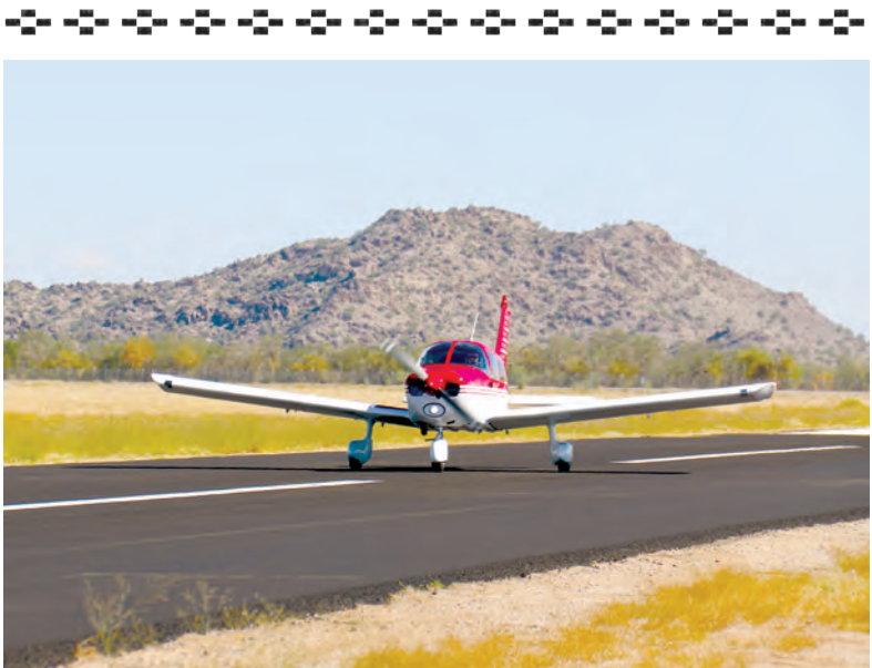
A small engine plane touches down on the newly paved runway at Ak-Chin Regional Airport.
