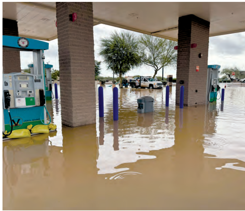
A submitted photo shows the gas pumps and parking lot of Vekol Market overflowing with rainwater.
