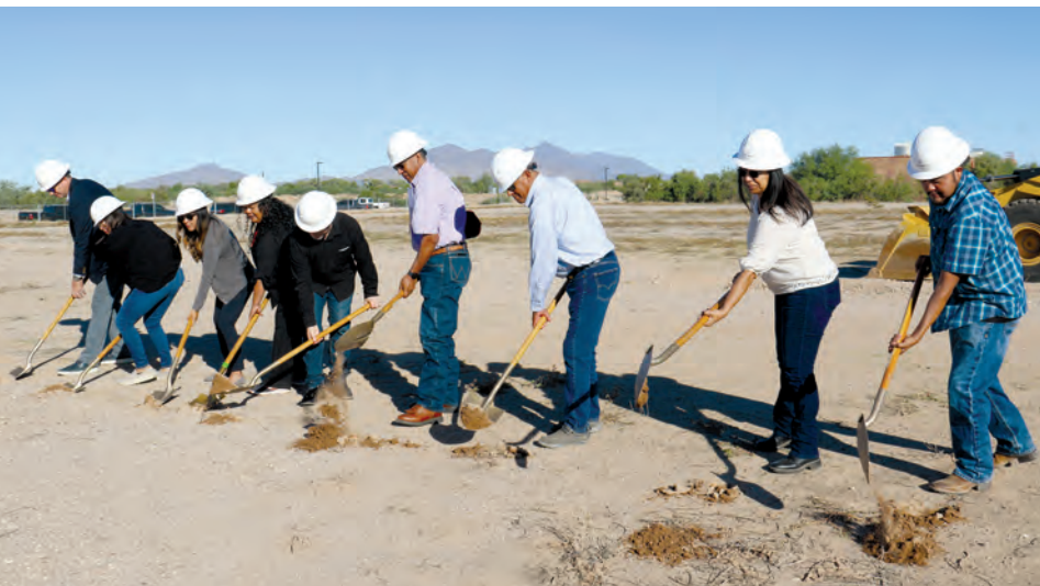
Members of the Ak-Chin Tribal Council, Ak-Chin Health Education Department and AR Mays Construction break ground on the Wellness Center.
