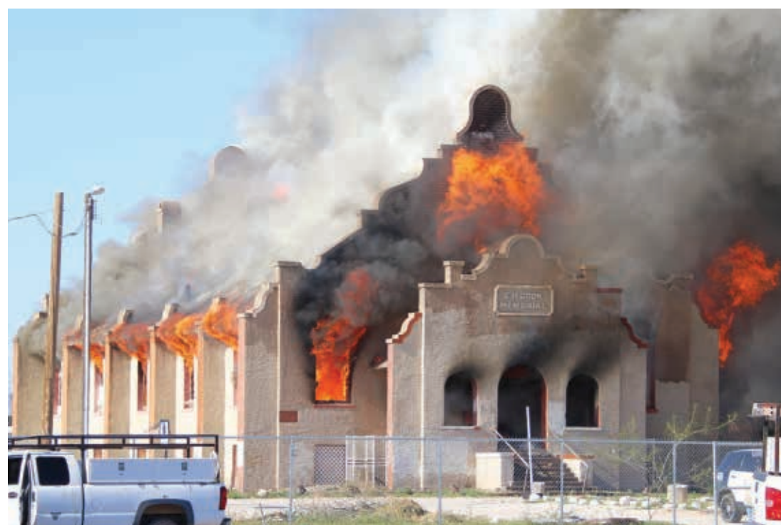
The C. H. Cook Memorial Presbyterian Church in Sacaton, built in 1918, is engulfed in flames on Monday morning March 25. The smoke could be seen ten miles away.
