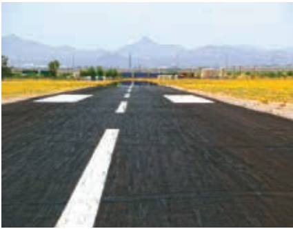
A plane's view approaching take-off on the newly paved runway at Ak-Chin Regional Airport.
