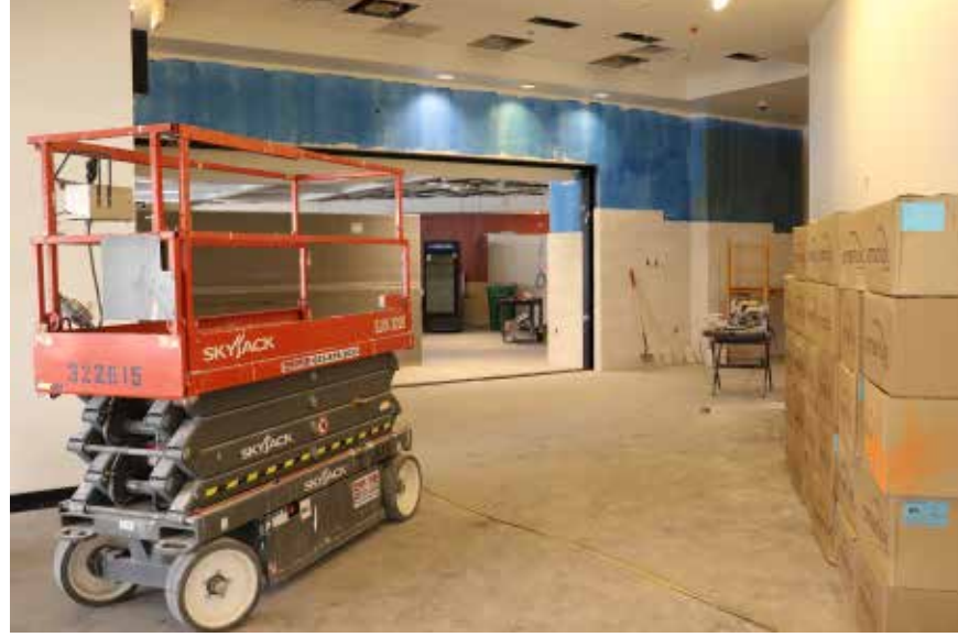
Progress in the hard hat zone outside of Agave's Restaurant.
